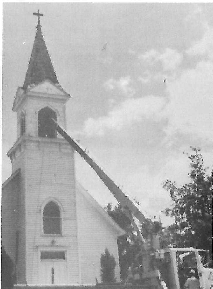
Removing bell from tower.
