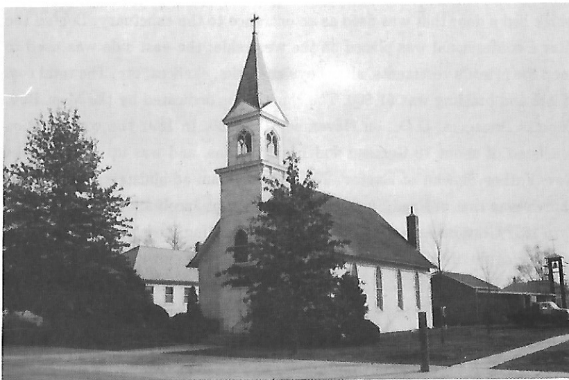
Old church and new rectory on the left.
