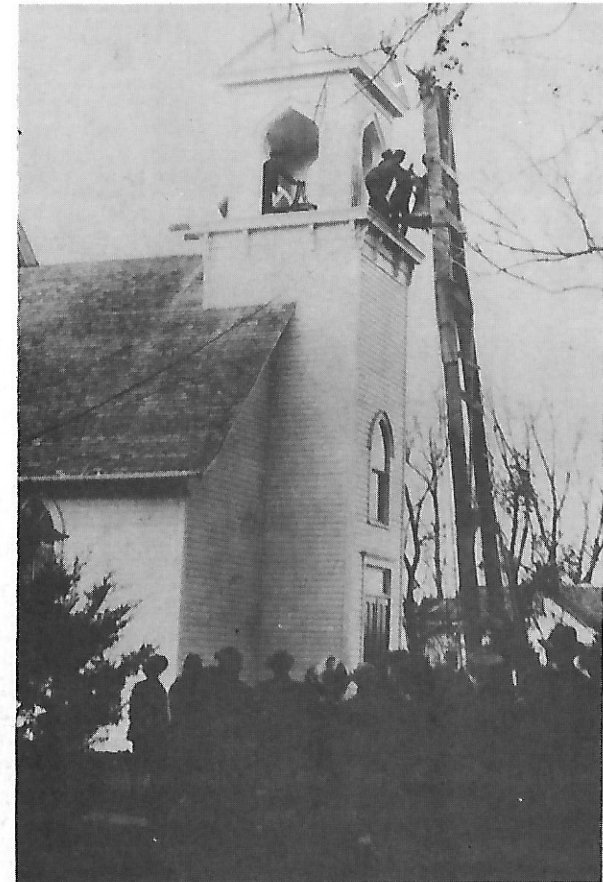
Installing Bell, Fall of 1912.
