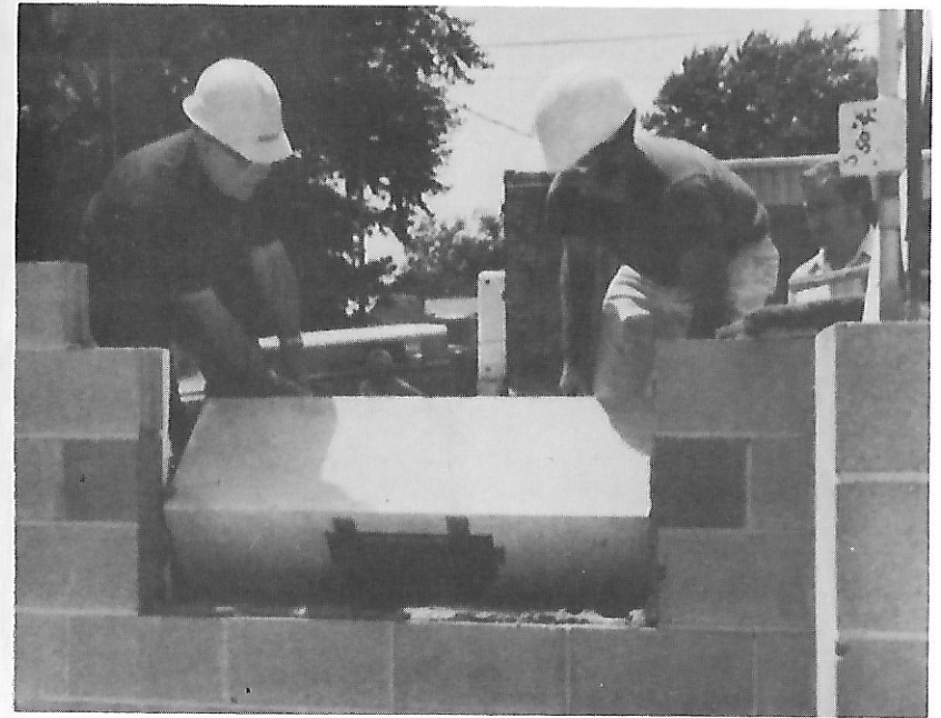
Workmen placing cornerstone.
